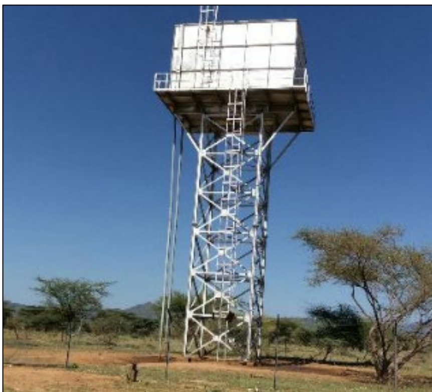
Figure 6.12-18: New Water Tank Linked to the Operator Piped Community Water System, Just North of Ngamia 1, Constructed 2018-19.
