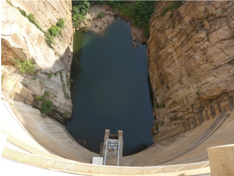
Photo 1: Plunge pool immediately below dam
