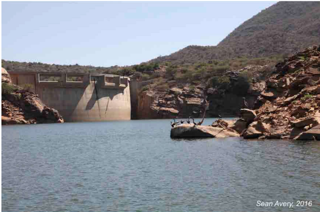
Figure 1: Turkwel dam (water level 28 metres below full supply spillway level)
