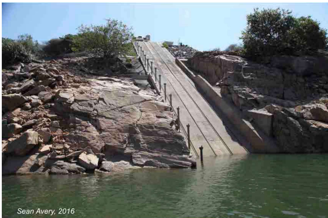
Figure 26: Intake screen maintenance ramp with water level gauges alongside
