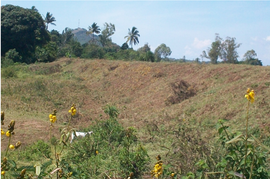
Plate 7.17: A dyke built to control flooding in Mukhobo Basin
