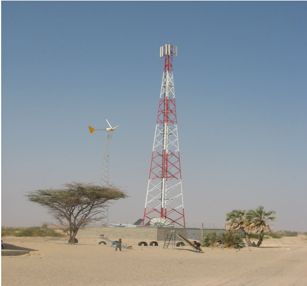
Plate 10: A Safaricom Limited BTS at North Horr. Note the harnessing of Wind Energy
