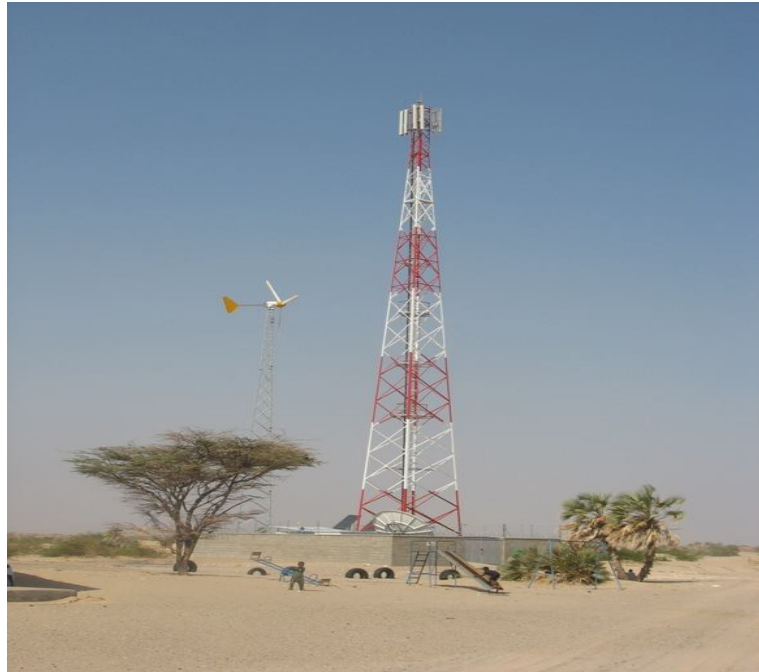
Plate 59: Harnessing of wind power (Note the windmill on the background used to power the transceiver)
