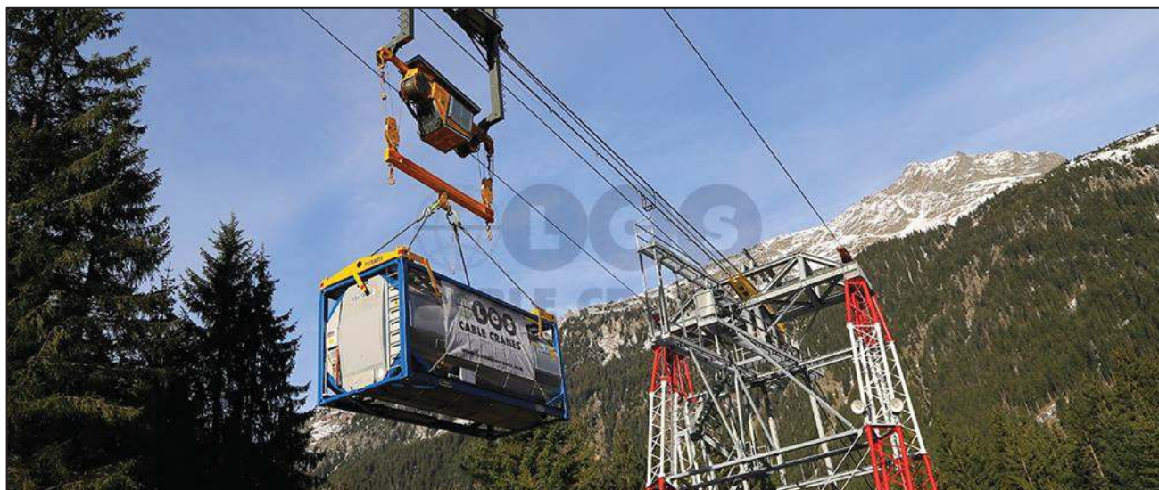
Figure 5.5-3: Cable Crane System for Water Pipeline Construction
