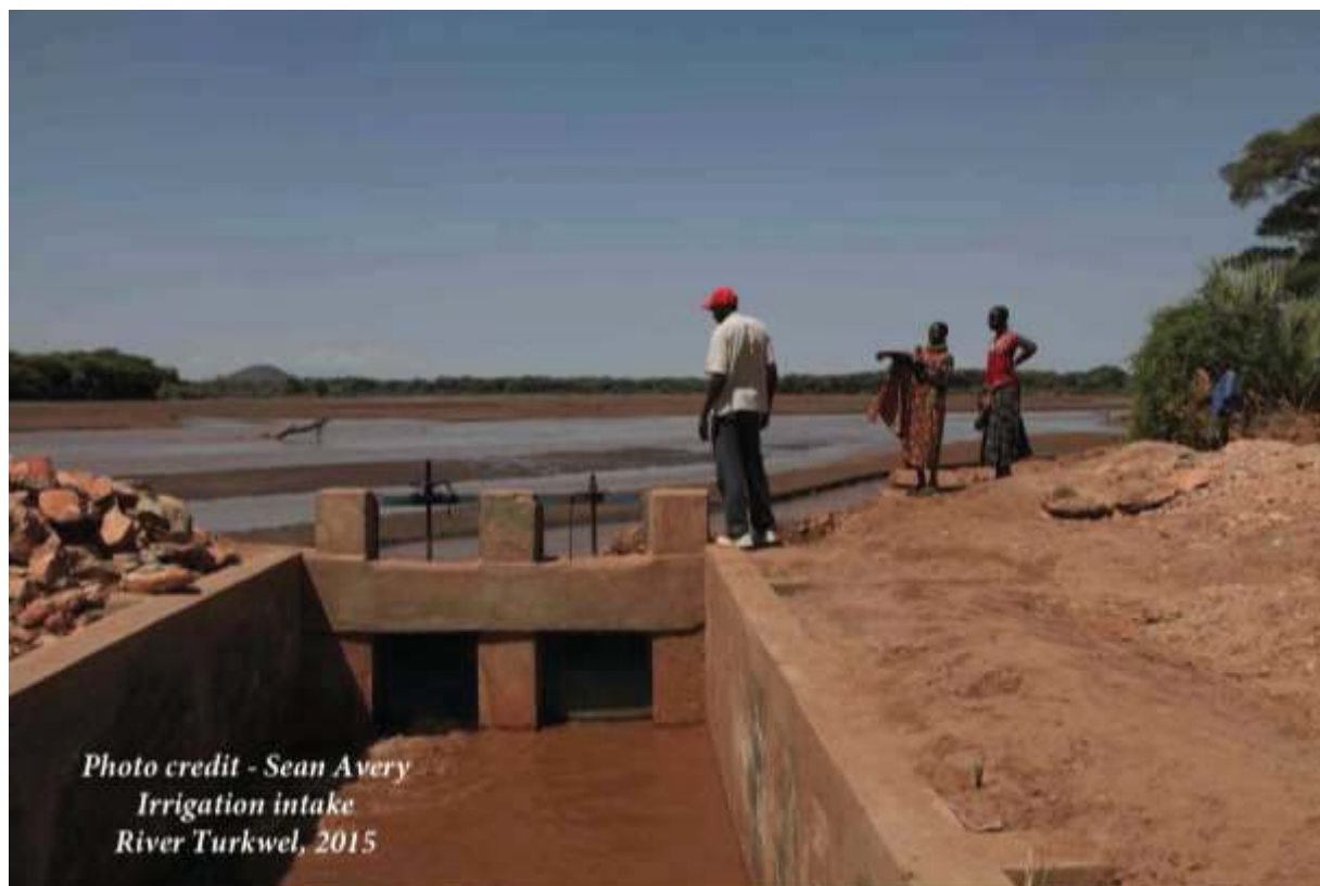
Figure 3: Irrigation intake from the River Turkwel (north bank of Turkwel)
