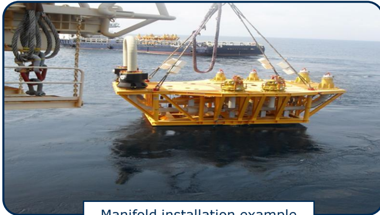
Manifold installation example
