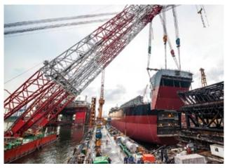
Turret block being lifted into position at front of TEN FPSO, during construction in Jurong shipyard, Singapore
